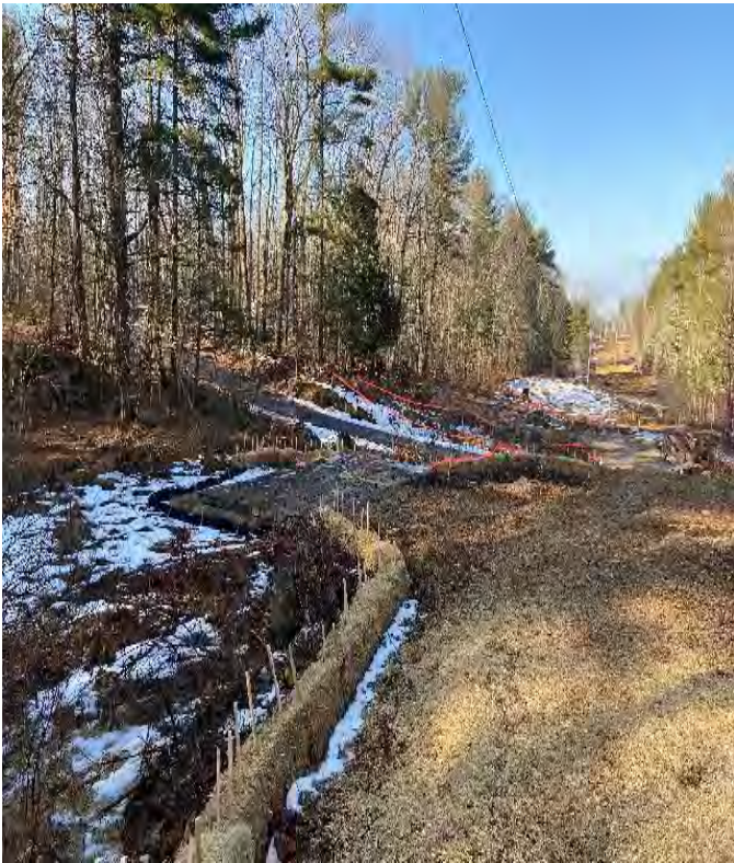
Fig 11: BMPs installed around wetland DW7 for work at Str. 63. Viewing west. (03-03-20).
