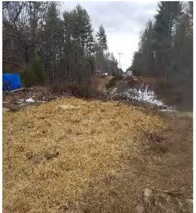
Fig 4: Straw spread over exposed soils at Str. 65. Viewing west. (03-02-20).
