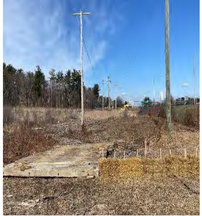
Fig 14: Str. 129 anchor point work pad. Viewing northwest. (03-03-20).
