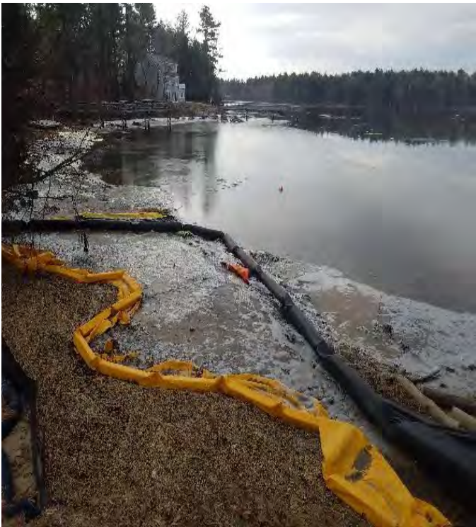
Fig 3: Turbidity curtain in intertidal zone at Gundalow landing/east side of the Bay. Viewing south. (03-02-20).
