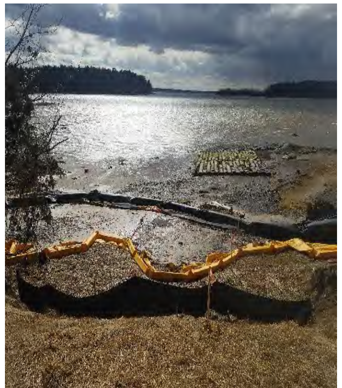
Fig 20: Turbidity barrier and concrete mattress at Gundalow landing/ east side of the Bay. Viewing southwest. (03-04-20).
