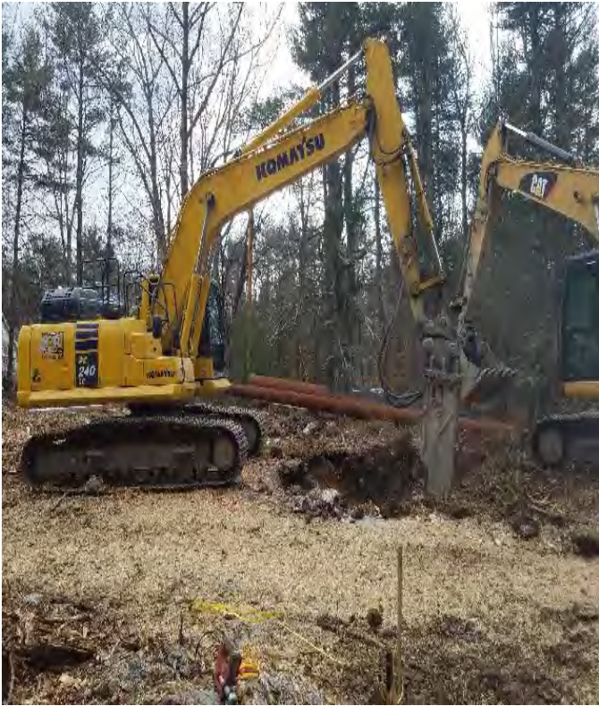
Fig 5: Beginning to excavate foundation for Str. 64. Viewing south. (03-02-20).
