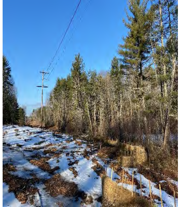
Fig 12: BMPs installed between Str. 62 work area and wetland DW5. Viewing northwest. (03-03-20).
