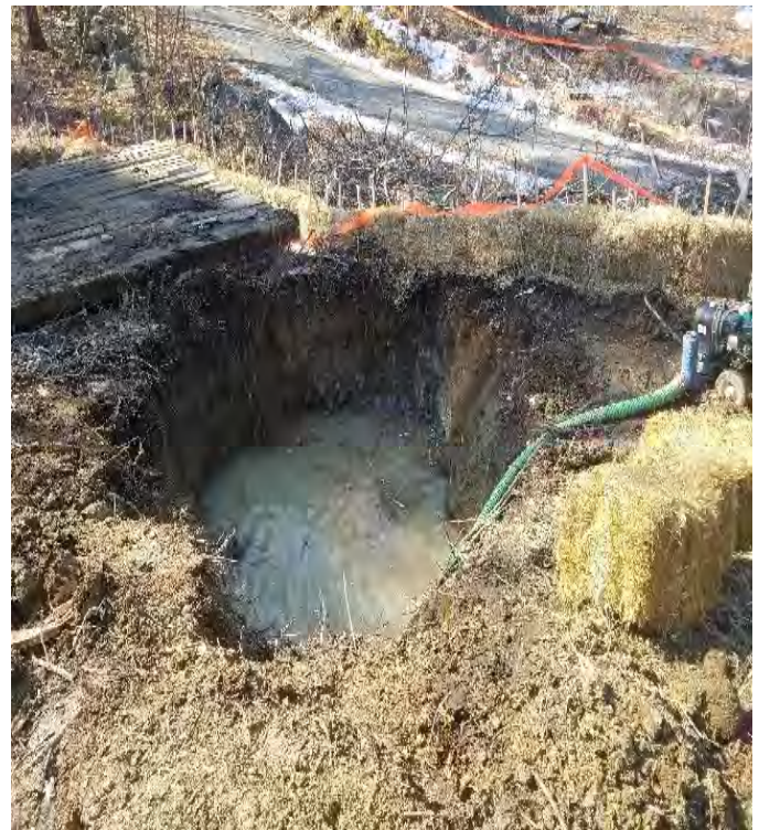
Fig 16: Pumping out water in hole at Str. 63. Viewing south. (03-04-20).
