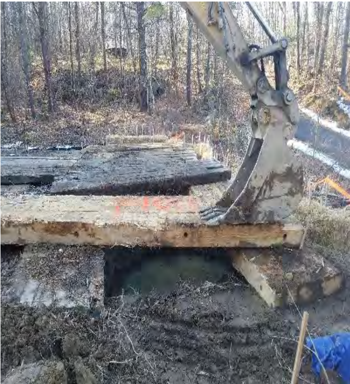
Fig 15: Groundwater in hole at Str. 63. Viewing south. (03-04-20).
