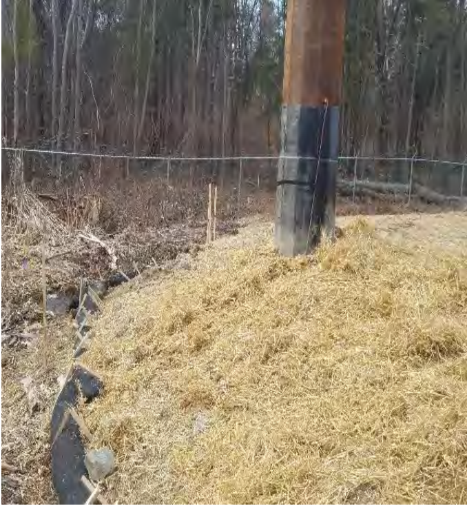
Fig 9: Str. 125 foundation. Viewing southwest. (03-02-20).
