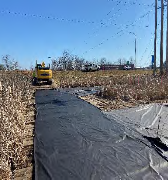
Fig 13: Installing filter fabric between timber mats at Str. 128. Viewing northeast. (03-03-20).
