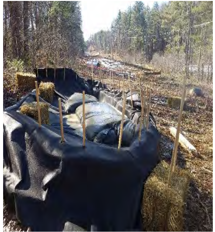
Fig 18: Pumping water from Str. 63 to dewatering basin. Viewing south. (03-04-20).
