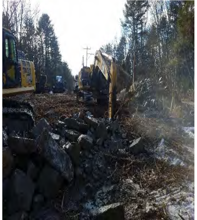
Fig 2: Excavating foundation for Str. 65. Viewing west. (02-28-20).
